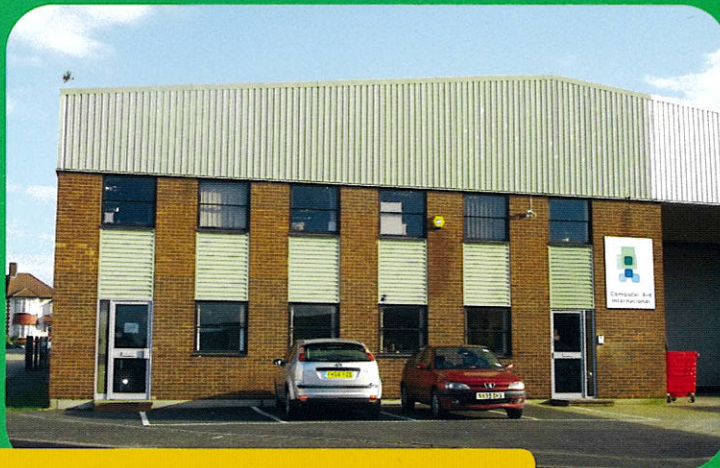
Computer Aid's new head office and warehouse in London, UK
