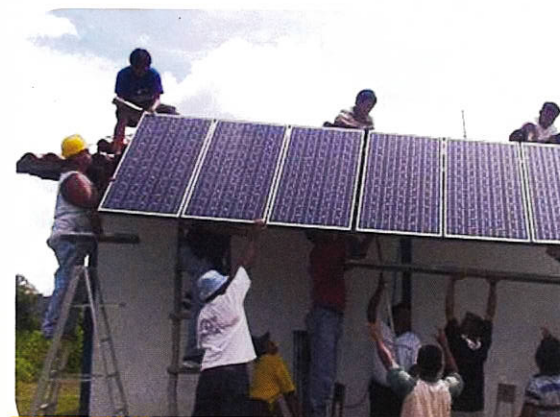
A solar panel is lifted onto the roof of a school, Venezuela
